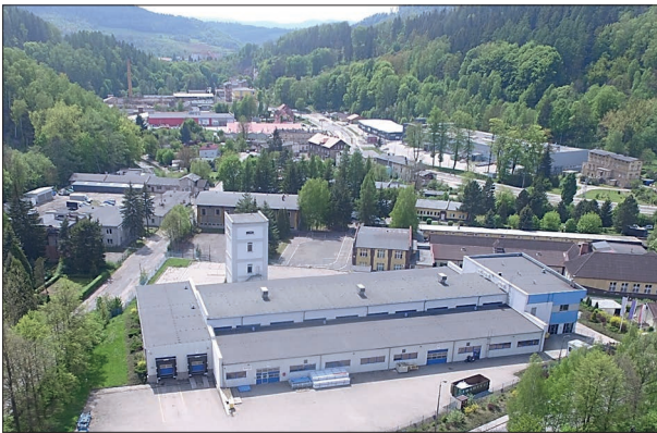
Nowa Ruda – Drogosław, Górnicza Street Outdoor Enclosures Production Plant
