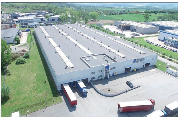
Nowa Ruda – Słupiec, Spacerowa Street Serial production plant and warehouse for finished products
