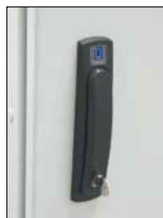
Lock with swing handle and cylinder insert
