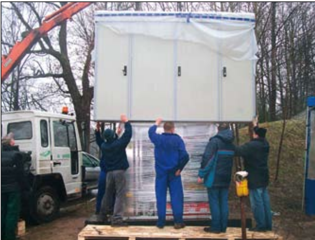
Cabinet during extension
