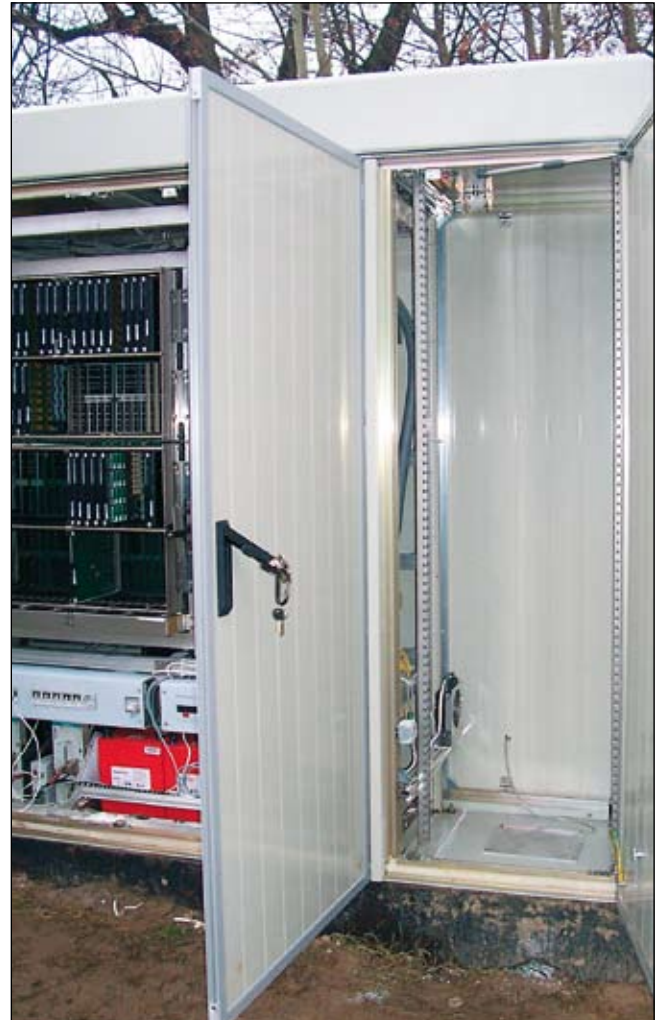
The Cabinet after extension
