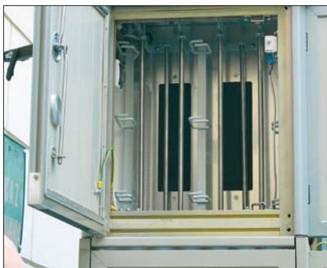
The Cabinet after extension
