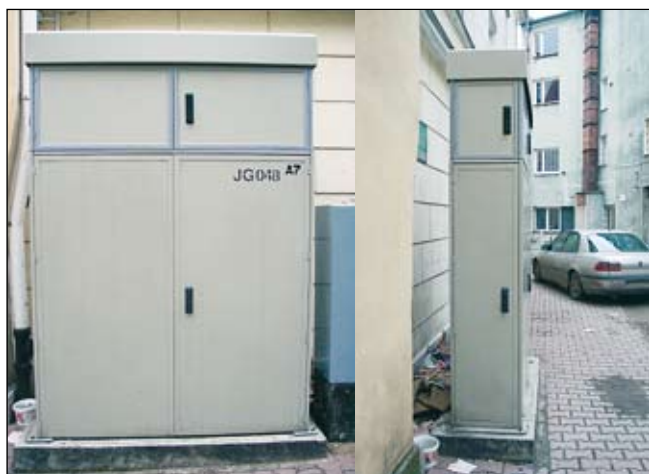
The Cabinet after extension
