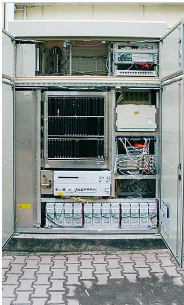
The Cabinet after extension
