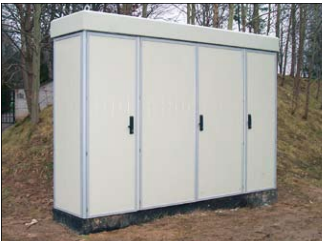
The Cabinet after extension
