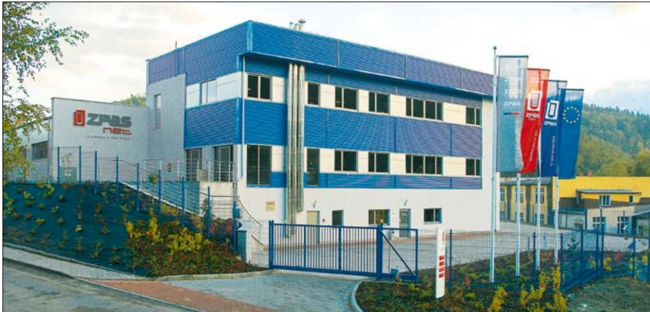
ZPAS-NET office building
