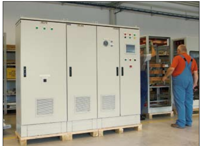
Assembly of power supply cabinets
