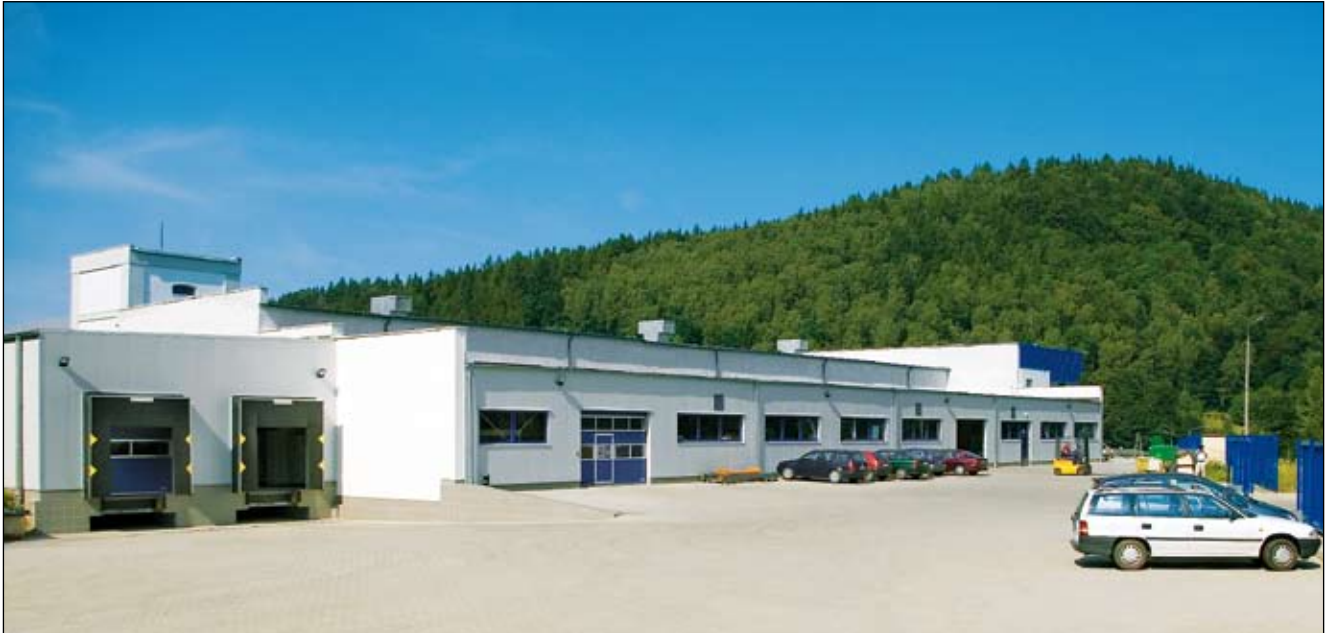
ZPAS-NET production facility
