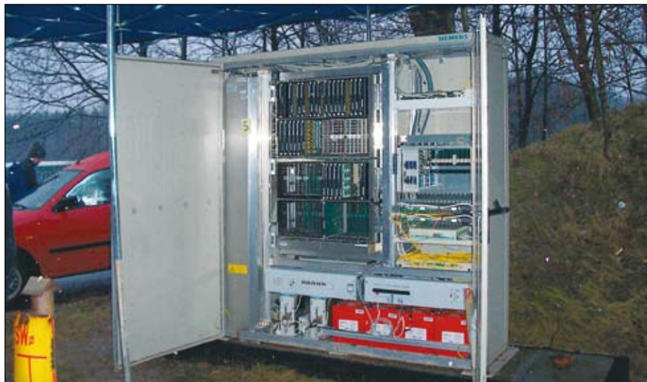
Cabinet before extension
