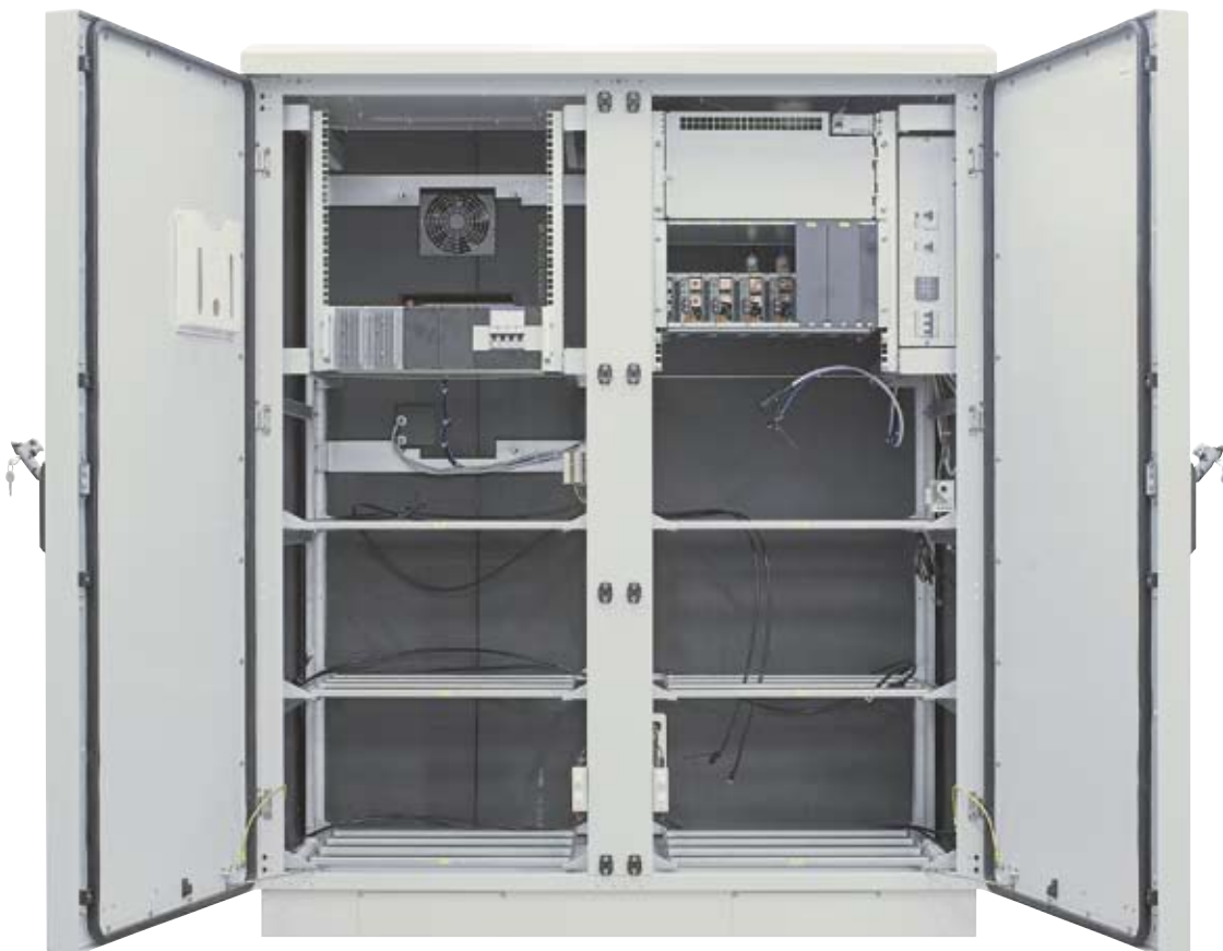
Cabinets completely made of aluminium sheet
