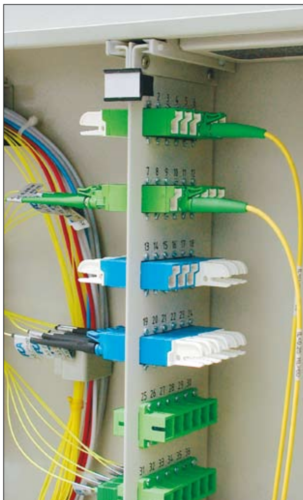
E2000 adapters mounted in OptiTel PSN distribution box (adapters and pigtails should be ordered separately)
