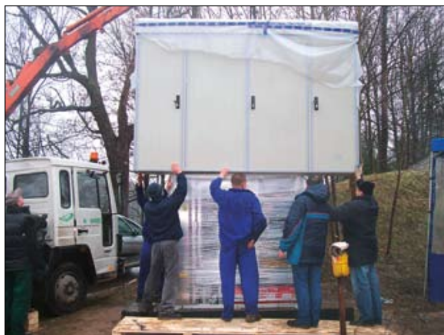
Cabinet during extension
