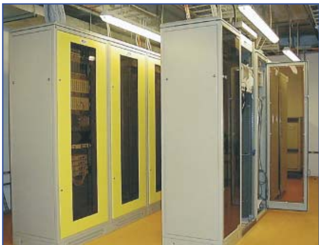
Main distribution room in Stock Exchange Warsaw building. The whole system is designed and manufactured on the basis of SZB cabinets. Installation done by ALMA SA. from Poznań (Poland) - http://www.alma.biz.pl
