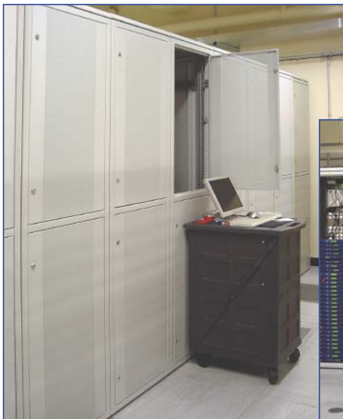
Collocation racks DSR installed in the internet server room by OVH in Paris (France).
