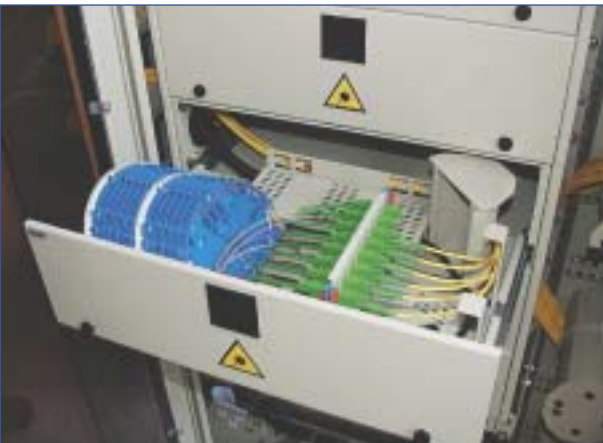
Connecting-commutation module MK-19/3U/72, with equipment
