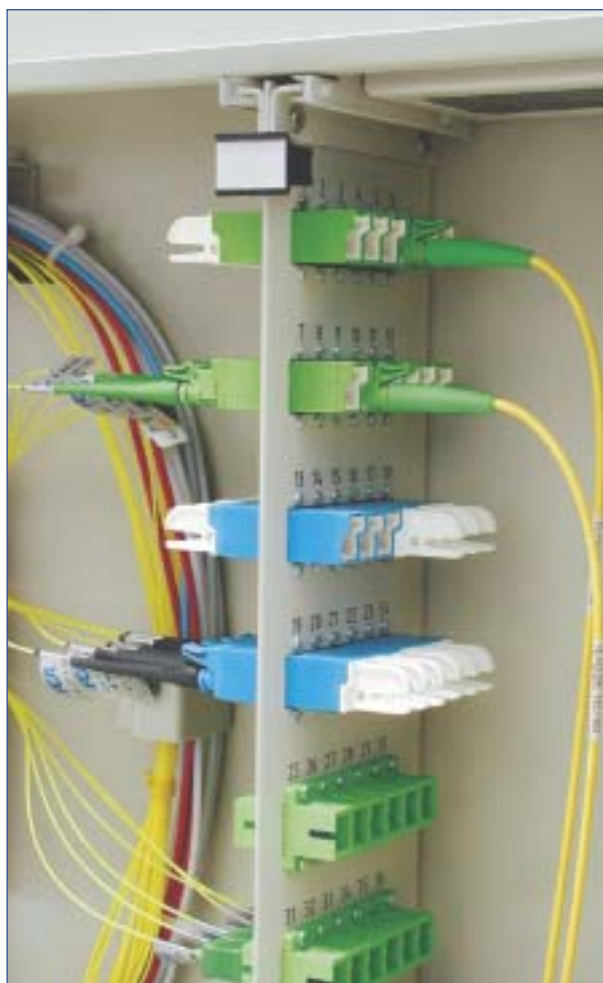
E2000 adapters mounted in OptiTel PSN distribution frame
