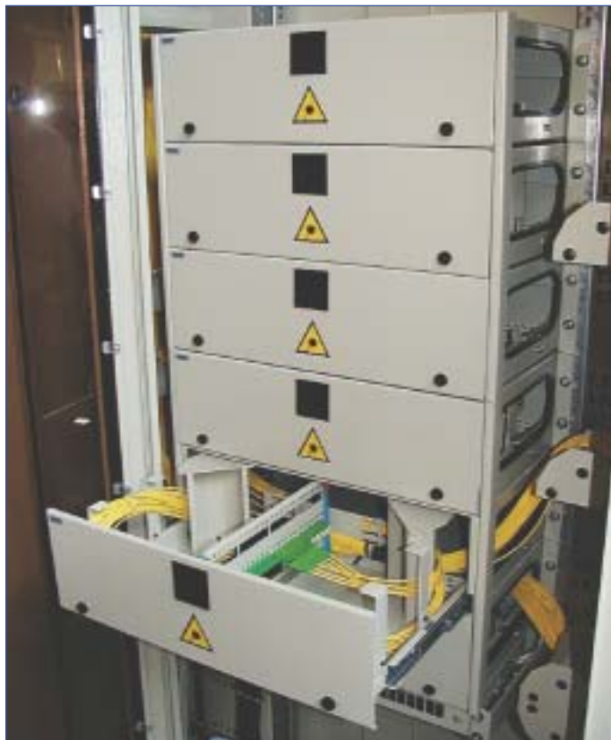
Commutation module MK-19/3U/72, with equipment
