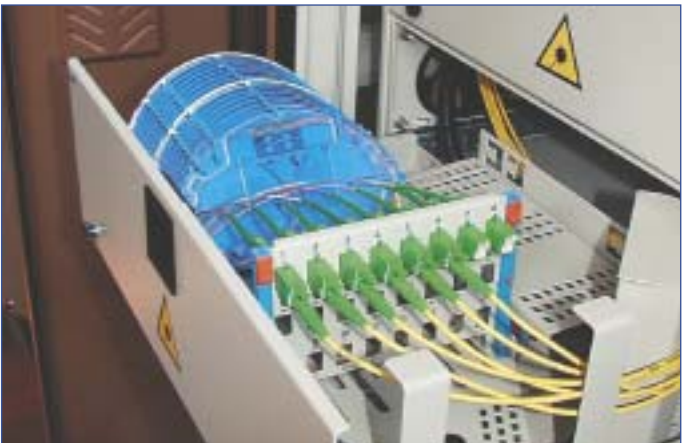
Connecting-commutation module MK-19/3U/72, with equipment
