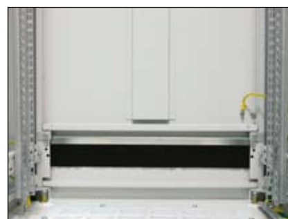
3 U module panel mounted in 600 mm wide cabinet
