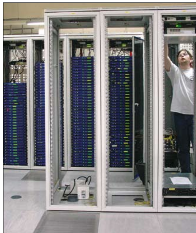
Installation of servers in SZB cabinets in OVH's internet server room in Paris
