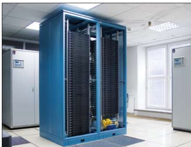
Collocation racks DSR installed in the internet server room by OVH in Paris France)
